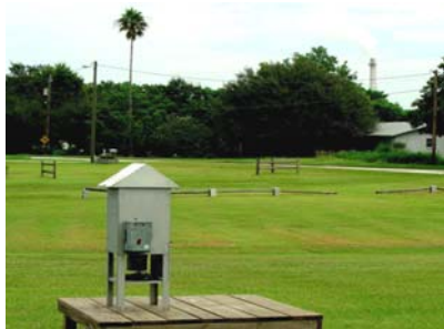
New air monitor located at Springhead fire station
