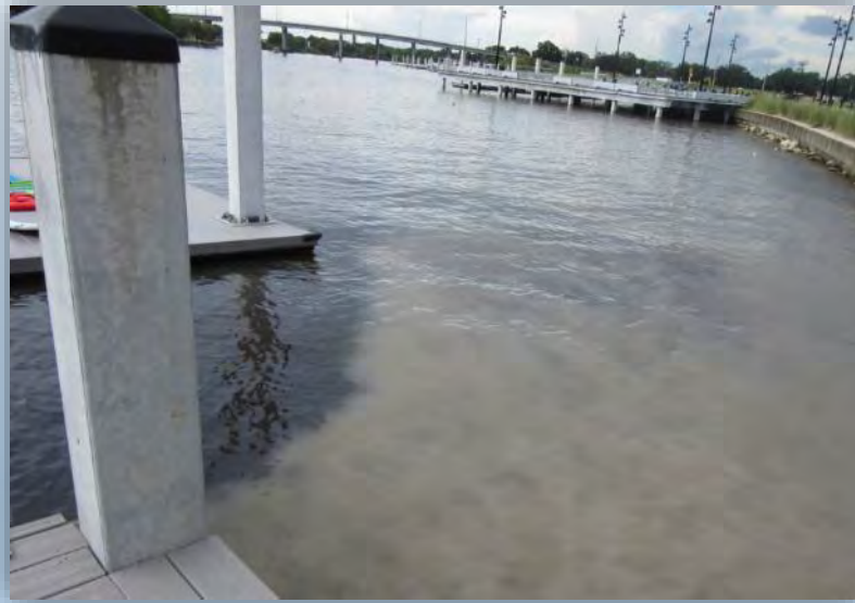
Downtown construction runoff to the River
