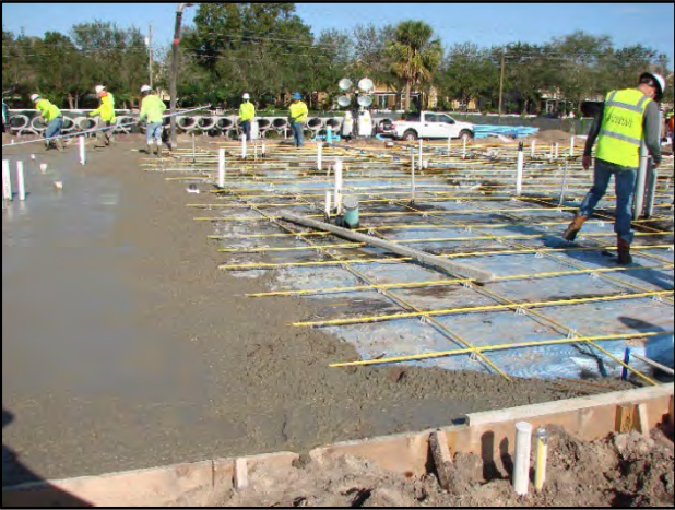
Above: Stormwater pond Below: Vapor barrier installation
