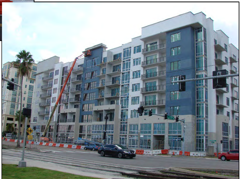
Above: Installation of auger-cast pilings, Spring 2022. Right: Construction progress Fall 2023
